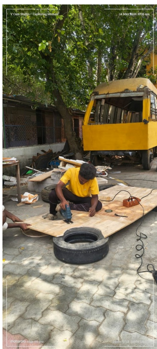
Cutting plywood for bus flooring and fittings
